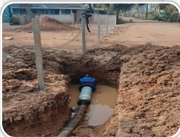
Replaced the 20 Years old pipe line with HDPE pipes at various underprivileged areas Kadiyam.
