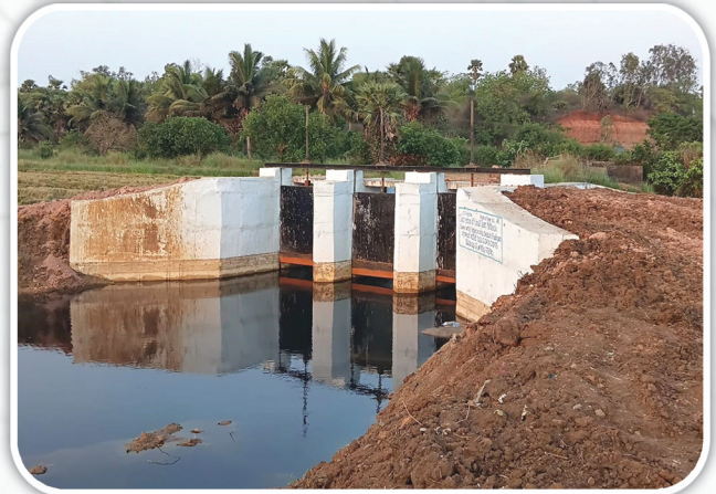
Constructed a small dam to block excess waterlogging in paddy fields during rainy season.
