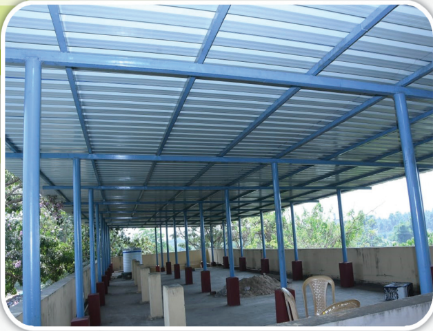
Constructed Sheds on Roof and at Entrance area to prevent water leakages at Community Health Centre Kadiyam.
