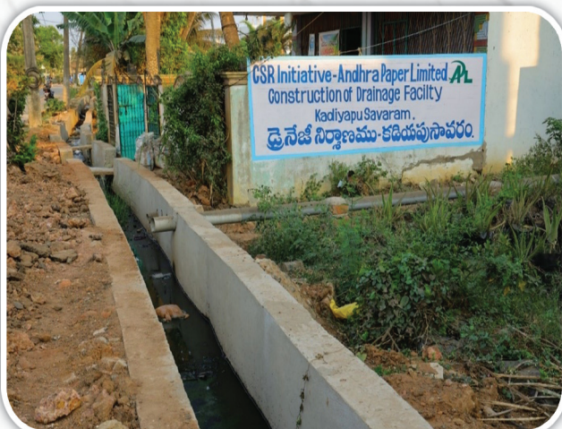
Constructed 500 meters of drainage adjacent to houses to prevent waste water accumulation at Kadiyapusavaram.
