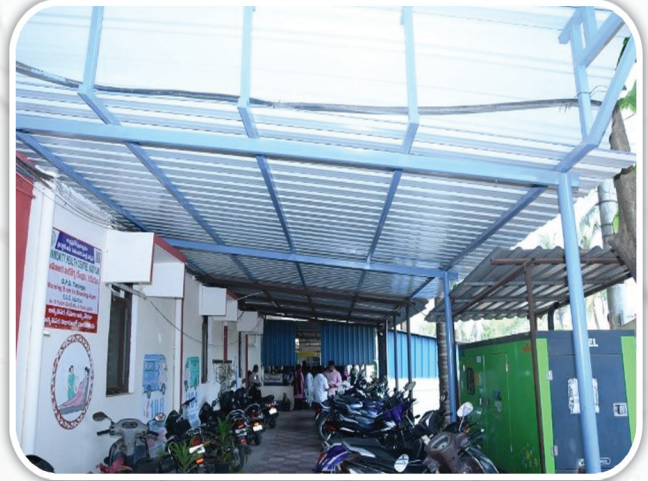
Constructed Sheds on Roof and at Entrance area to prevent water leakages at Community Health Centre Kadiyam.
