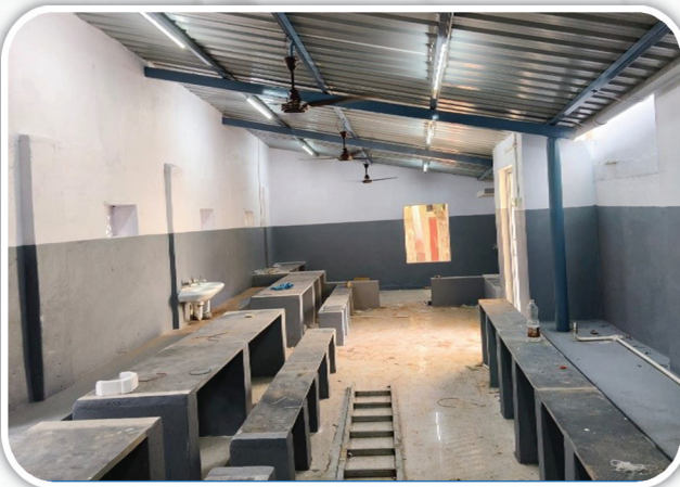
Constructed a Dining Hall at MPP School Veeravaram.
